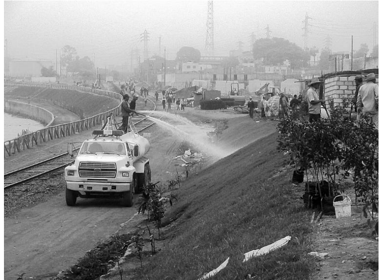
Figure 2 Irrigation of green areas by lorries using drinking water.
